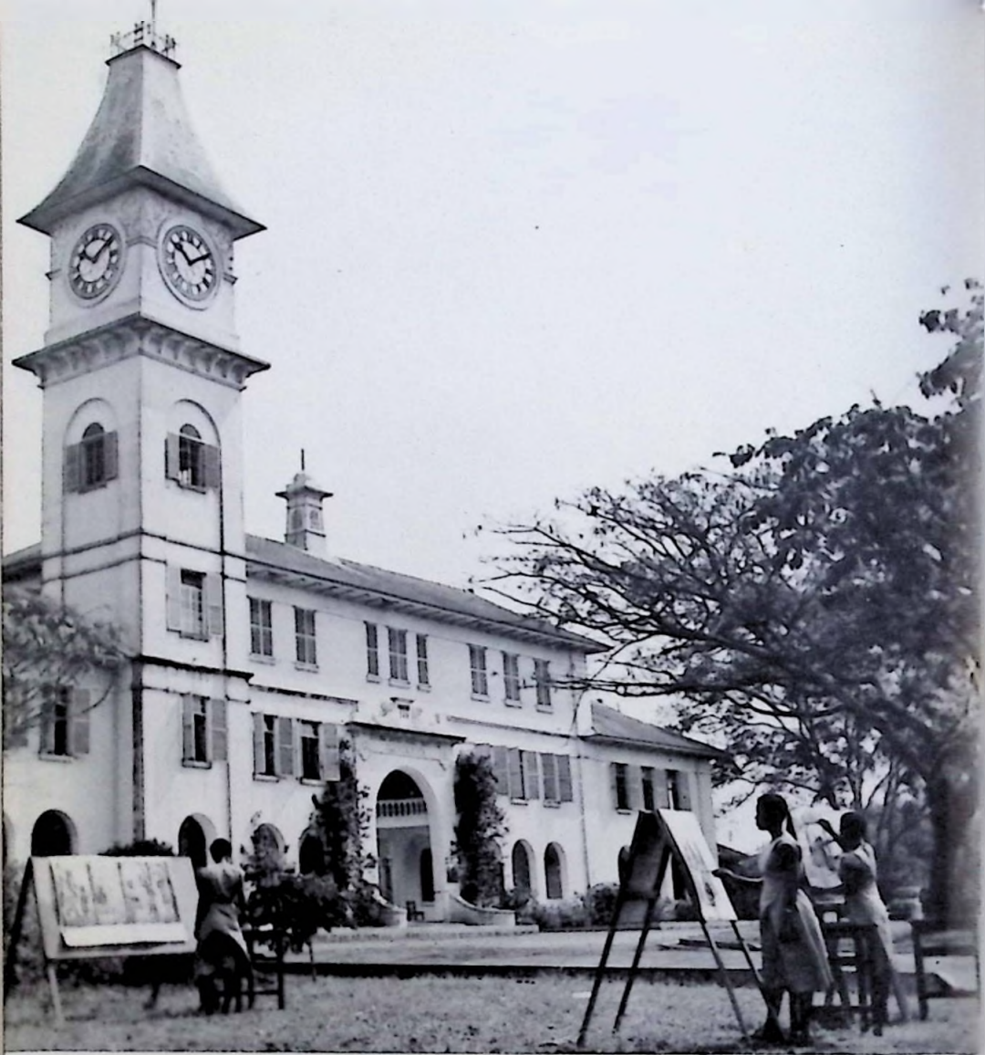
The Administration block
