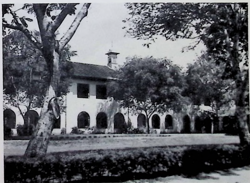
West classroom block
